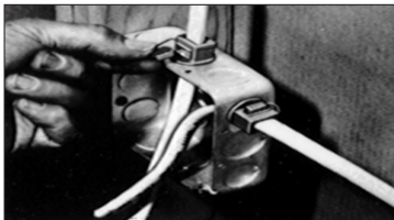
Snap captive locking wedge into connector's cavity.
