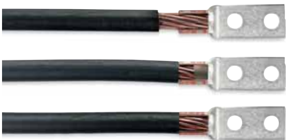
Strip Length Too Long
