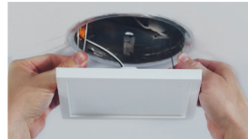
Torsion springs for recessed housings
