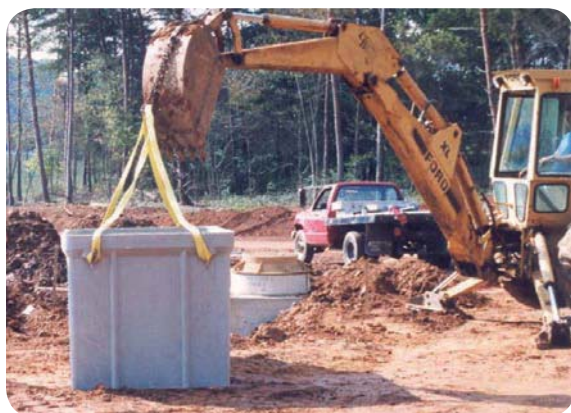
Lift and position enclosure with backhoe.
