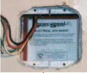
When used within metallic switch and receptacle boxes, inserts are UL Tested and Classified to permit larger boxes and reduced spacing.
