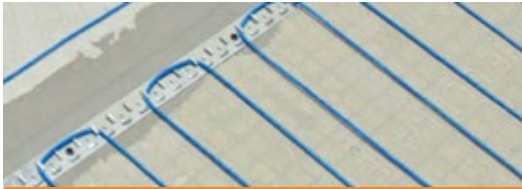
WarmWire installed using CableStrap
