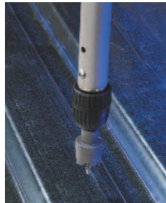
2. Drill Deck Holes
