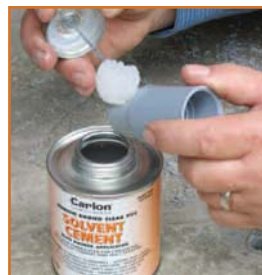
Apply a uniform coat of cement.
