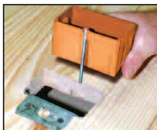
Install clip over subfloor.
