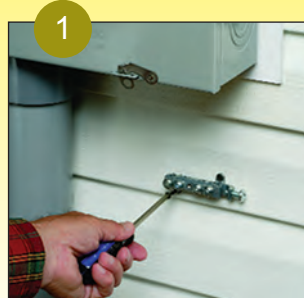
1 Attach bridge to substrate. (Mounting screws not provided.)
