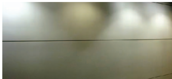
This is an example of an application where tight color specifications were not met.
