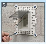
Install NM cable connector and wire. Attach recessed IN BOX to block. Holes in flange allow stucco to bond firmly.
