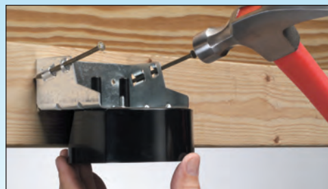
Nails to SINGLE JOIST
