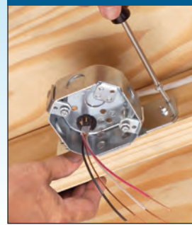
FBS415S/FBS420S Mount on SIDE of Joist
