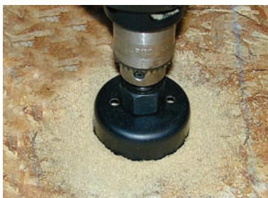
2. Drill hole in floor using hole saw.
