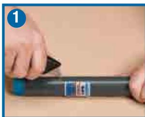
**Step 1** consists of two cuts through the plastic to the substrate along the length of the conduit, approximately ½" apart and 3" to 4" in length. A third, perpendicular cut crosses the lengthwise parallel cuts.
