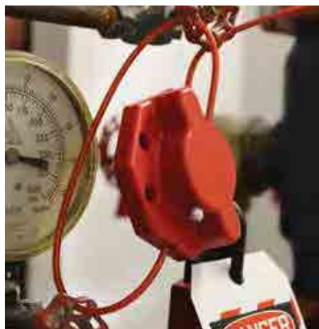
Turn the hasp halves to cinch cable.
