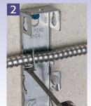
Bend tab over the cable, locking it securely in place.
