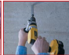
2. Snap on drive sleeve and drive in anchor
