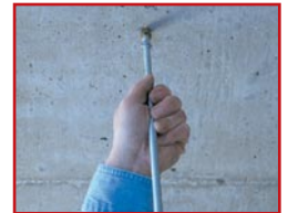
3. Insert threaded rod
