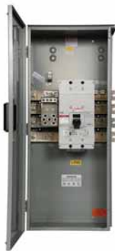
Main Circuit Breaker
