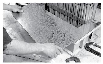
Intumescent sheet used to firestop large openings. Designed to seal penetrations against flame spread, smoke and toxic fumes. This composite sheet has multiple applications, including blank openings, through penetrations of multiple cable, pipe ducts, buss ducts and cable trays.
