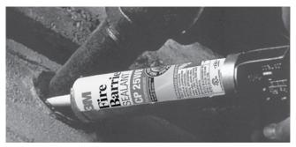
All 3M Fire Barrier Sealants have either intumescent, endothermic or ablative technologies designed to provide a tight and dependable seal against fire, smoke, toxic fumes and moisture. 3M intumescent sealants expand up to 10 times their original size when exposed to temperatures over 300°F (149°C). This intumescent action forms a strong, insulating char that seals the opening for up to four hours when exposed to extreme heat.
