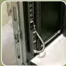
Power Distribution & Surge Protection
