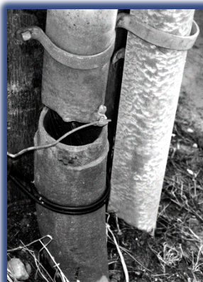
Steel U-Guard required grounding, strapping, and does not have belled ends.
