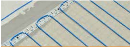
WarmWire installed using CableStrap
