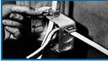
Snap captive locking wedge into connector's cavity.
