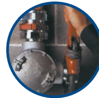
5. Install hub on enclosure
