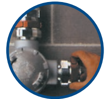
6. Insert cable and tighten red union
