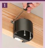
Install FBA426 onto joist with (4) screws: (2) through support tabs A and B, and (2) more through the front flange.
