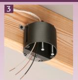
Pull NM cable through installed NM connector.
