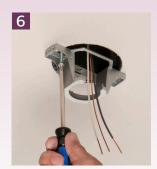
Box flush with ceiling. Remove captive installation screws and install bracket.
