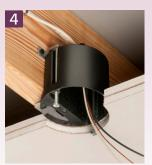
Cutaway: Box set back in double drywall ceiling.
