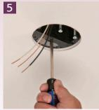
After installation of wall board, use the depth adjustment screw to adjust position of the box, if necessary.
