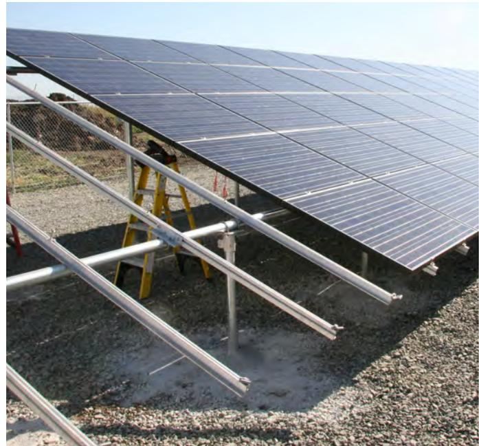
*This is a U-LA installation using SolarMount beams and clamps. Designed and installed by Minyard Solar*
