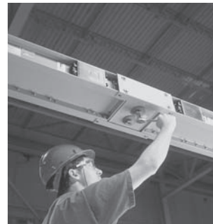
Typical Busway Installation (Torque Indicating Bolt)
