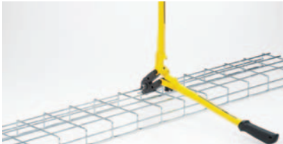
4 Turn tray open-side down and cut wires from bottom of tray.
