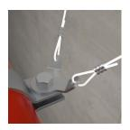
• Attaches cable brace to structure
