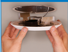
6-inch friction clip position
