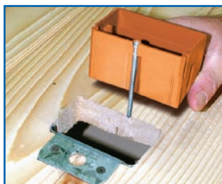
Install clip over subfloor.
