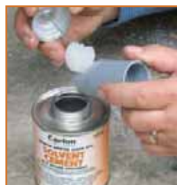
Apply a uniform coat of cement.
