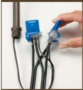
Hold wires in place while squeezing handles together until the connector snaps shut
