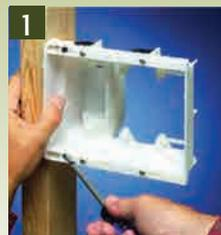
Attach box to stud. Use tabs for proper positioning of box depth. See 2.
