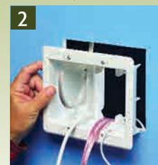
Attach trim plate to box. See Photo B. Pull wire/cables. Install box assembly in opening.
