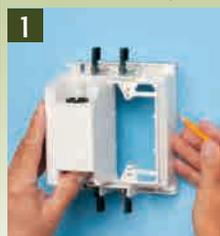
Using box, without trim plate as a template, mark location. Cut hole.
