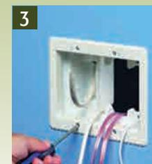
Tighten mounting wing screws to pull the box securely against the wall board. See Photo B.
