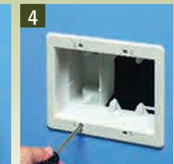
Tighten mounting wing screws to pull the box securely against the wall board. See Photo B.
