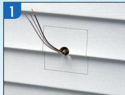
Disconnect electrical power. Place box section in desired location and pencil outline onto siding.
