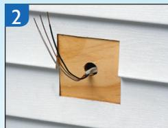
Cut along pencil line with razor knife and remove vinyl siding.
