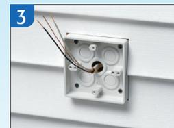
Mount box section to substrate. Caulk as required.
