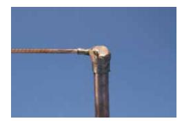
The reaction produces a finished permanent exothermic connection
