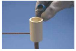
Position CADWELD ONE SHOT and wire on prepared ground rod. Dump the welding material into the ceramic crucible.
