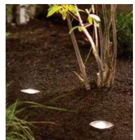
In-Ground Lighting with LED
