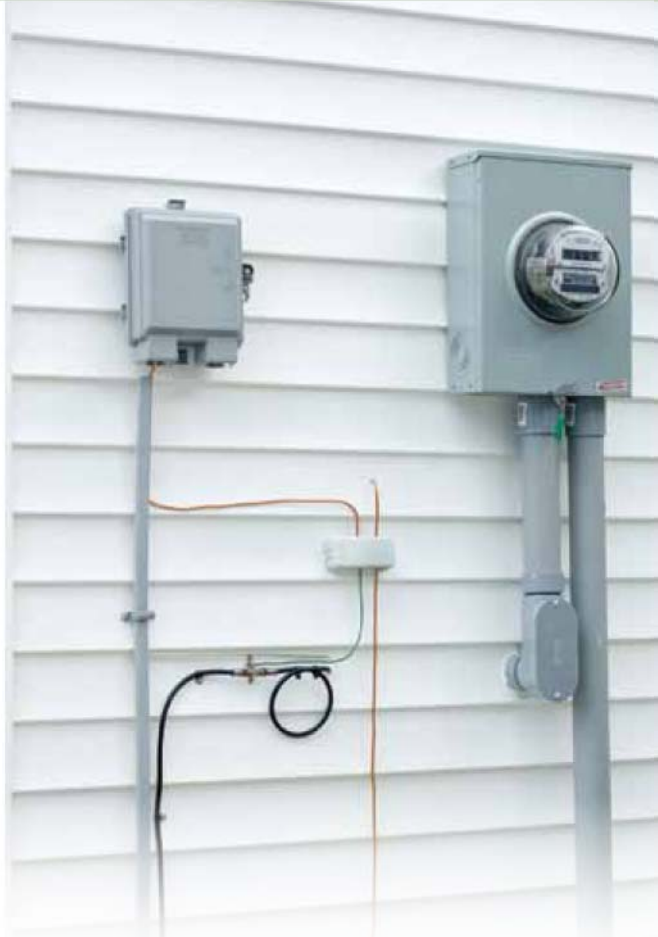
Intersystem Bonding Termination Bar (IBTB)
