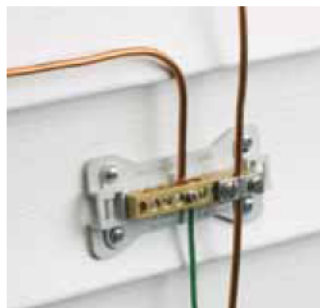
Intersystem Bonding Termination Bar (IBTB)
