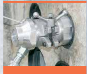
Complete the assembly and blow in tape.
