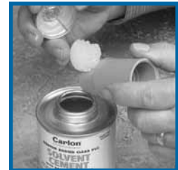
Apply a uniform coat of cement.
