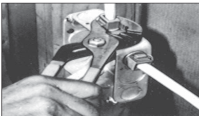
Press locking wedge into cavity which locks onto cable.
