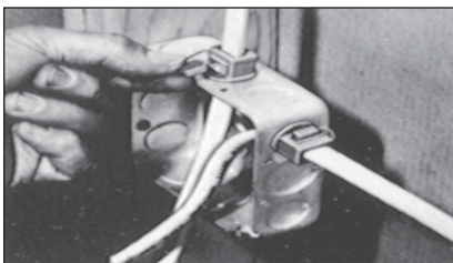
Snap captive locking wedge into fitting's cavity.
