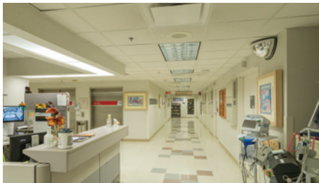
Before: Fluorescent Lighting
