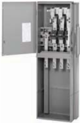
Main Fusible Switch with Utility Pull Box
