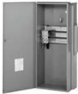
Main Terminal Box
