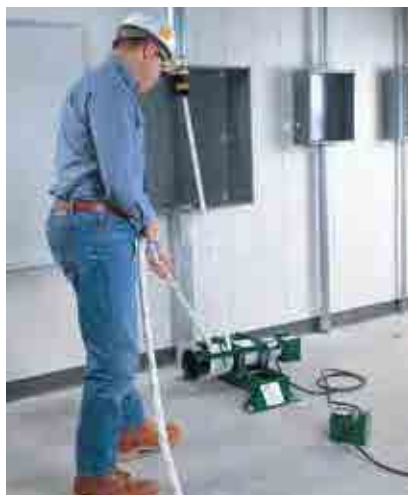
Operator is making a downward pull from the box using the puller with the floor mount anchored to the floor.
