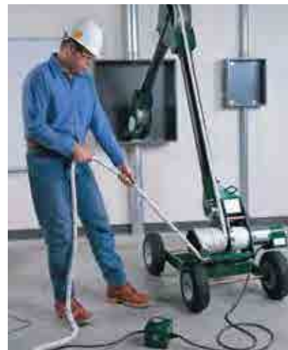
Operator is making an upward pull from the box using the puller and Versi-Boom Plus System attached to the mobile carriage.
