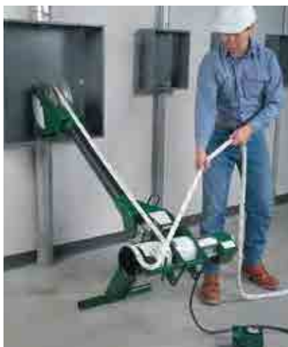
Operator is making an upward pull from the box using the puller and Versi-Boom System attached to the "T" stand.
