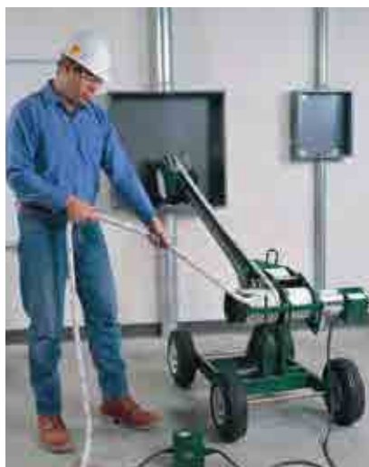
Operator is making an upward pull from the box using the puller and Versi-Boom System attached to the mobile carriage.
