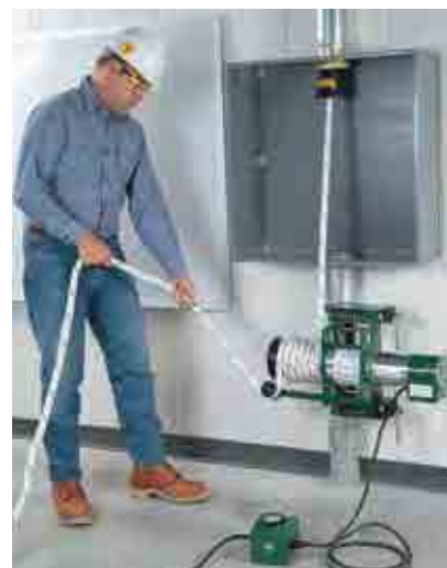
Operator is making a downward pull from the box using the puller with the chain mount (or vise chain unit) mounted onto the conduit.
