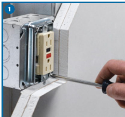
1 Loosen... The two adjustment screws located on opposing corners of the mud ring.
