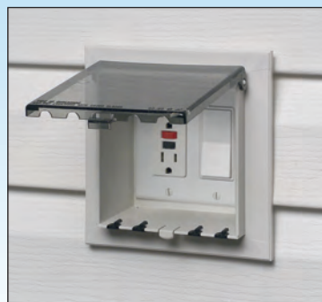
Completed installation, DBVS2C shown.
