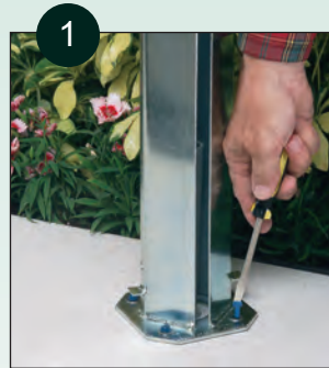
1 Metal support post attaches easily to surface.
