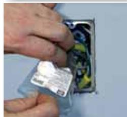
Tighten mounting screws, attach wallplate and trim out complete.
