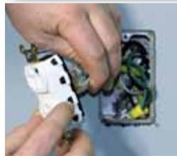
Remove protective packaging. Snap the duplex to the circuit.
