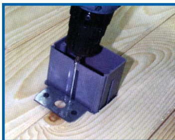
Screw in to adjust to height of flooring or carpet
