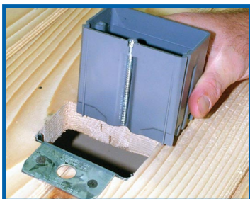
Install clip over subfloor.
