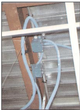
ENT and Carlon boxes roughed-in for fixture whips
