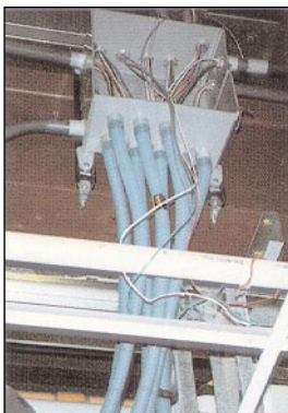
ENT above a suspended ceiling for receptacle drops
