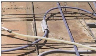
Stub Down Using Carlon's PV Mold
