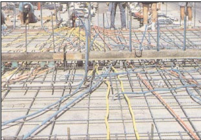
Carlson ENT roughed-in a deck (between layers of rebar) ready for a concrete pour (tunnel form).
