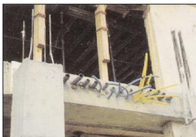
ENT in a Floor Slab prepared for more form work to extend conduits in the next pour.
