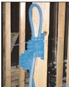
Wall Box Installation.
