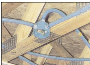
Carlon Ceiling Box and ENT roughed above a ceiling.
