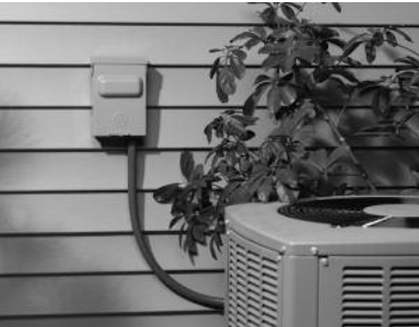
As an air conditioner disconnect
